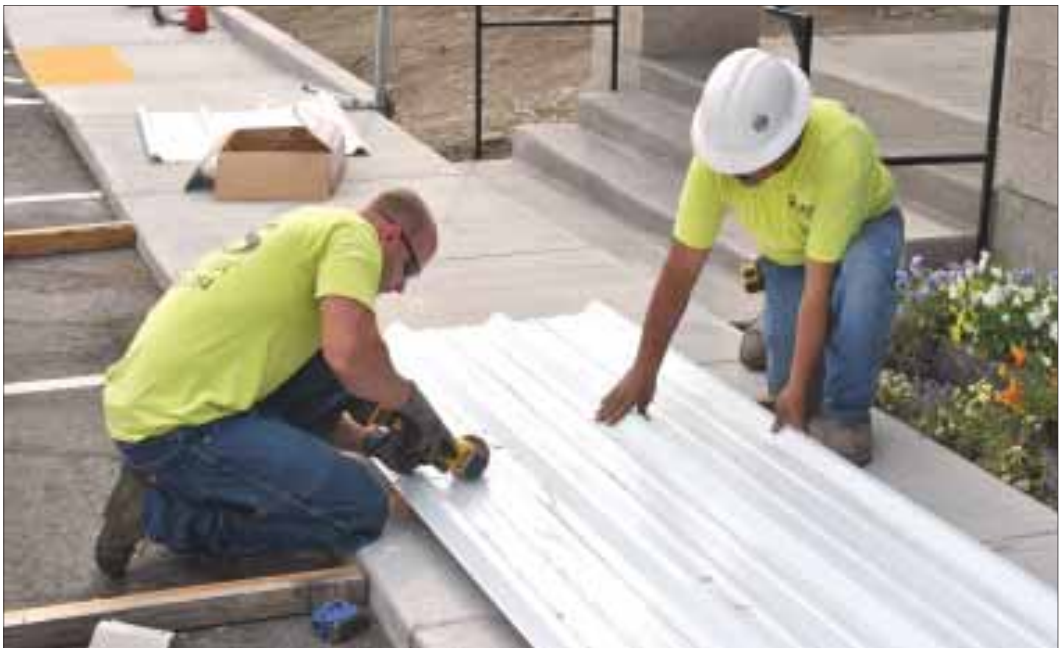
Above: R & S Constructors crewmen put the finishing touches on a metal panel. Below: New Gypsy Jackson librarian Karine Parry welcomed patrons back to the library Friday.
