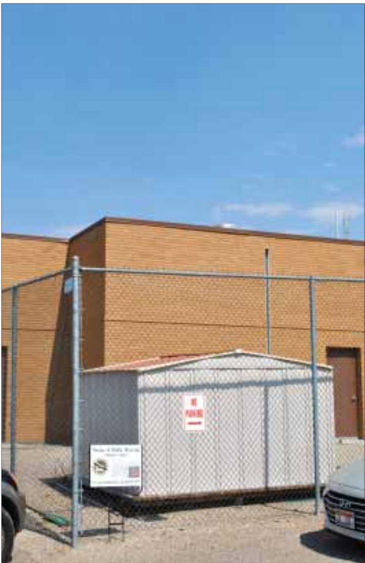
The proposed tower for the broadband project will replace this shed behind the Owyhee County Courthouse in Murphy.
