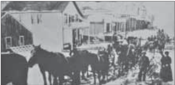
Silver City in early 1900s (after construction of Swan Falls power plant and a line to the town.)
