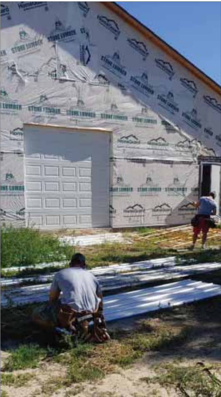
Stucco, siding and painting were accomplished in one of the biggest days of finish work at The Rock of Homedale late last month. Submitted photo
