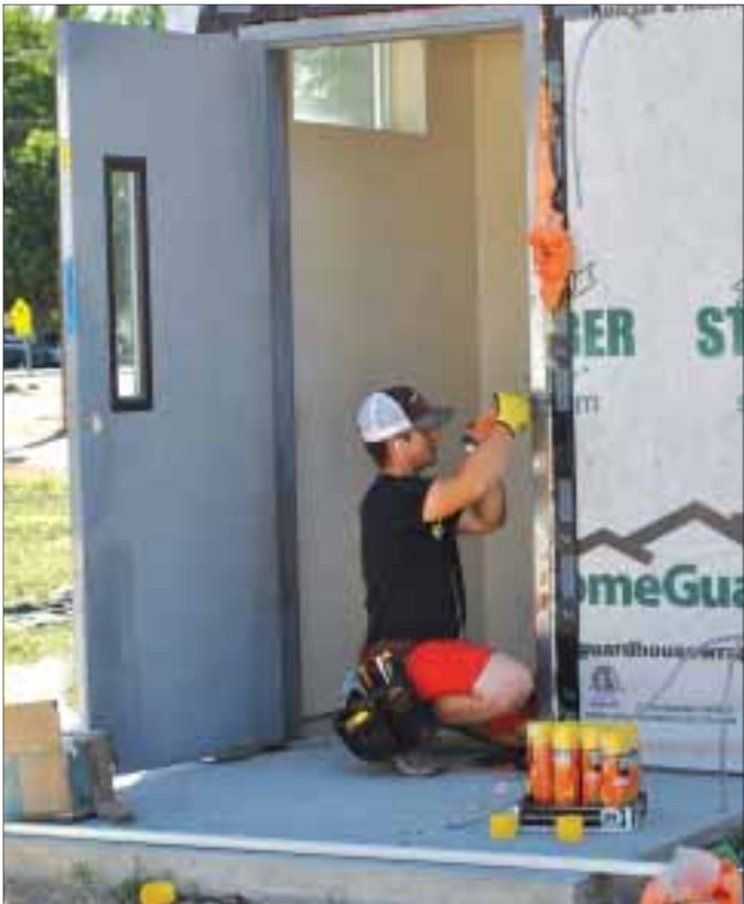
Work on local youth refuge inches along Ideal Construction's Drew Deal puts in some work on Thursday at The Rock of Homedale youth center on East Wymoning Avenue in Homedale. Donations for The Rock can be made at www.therockofhomedale.org .
