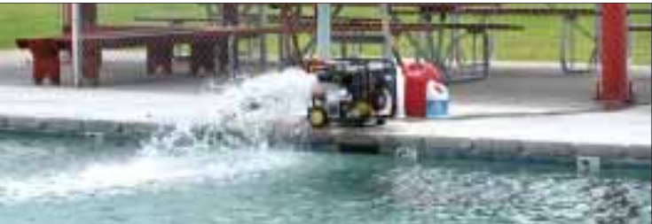
A surface pump used last week to keep city pool water circulating while the primary pump was repaired.
