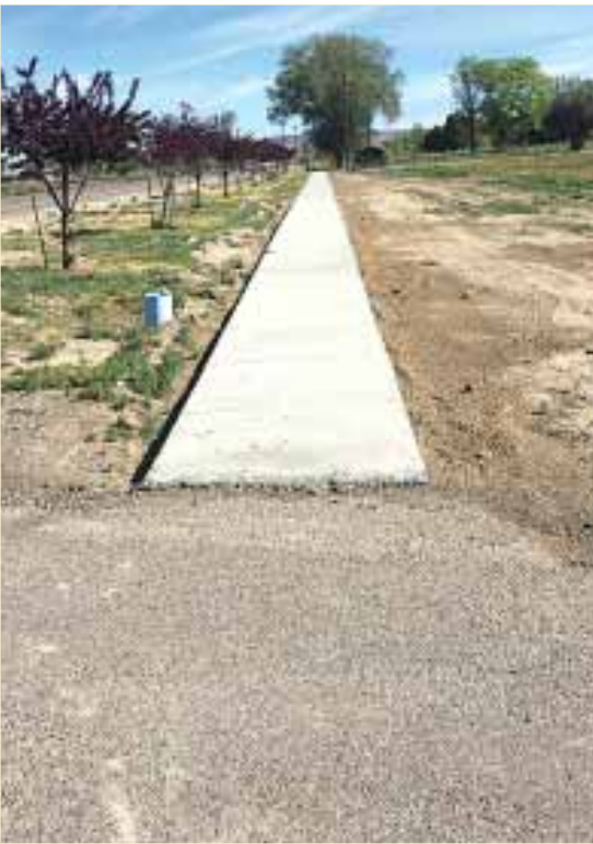
The final 380 feet of concrete has been placed in the Grand View Greenbelt. Submitted photo
