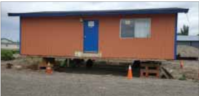
County annex shapes up in Grand View The building to house Owyhee County’s Grand View substation, which would include both Division of Motor Vehicles and sheriff’s office services, has been in place since June 5. Work began this week. Photo by Mandi Boren
