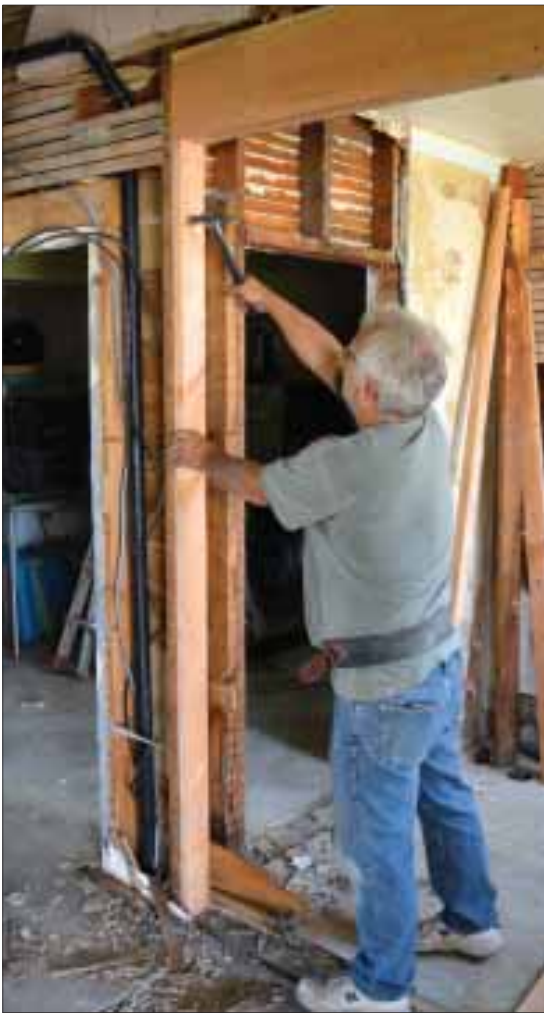
Mike Platt, from HCD, Inc., pounds down some nails near the front entrance to the new Marsing City Hall, formerly The Sandbar Restaurant with a Cause.
