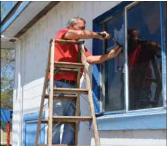
Marsing bus barn vandalism repaired Bill Jones, of Nampa’s Jones Glass, uses a hammer and screwdriver to delicately remove tape from a window on the south side of the Marsing School District transportation building. Jones and his crew replaced windows that three vandals — identified by Owyhee County Sheriff’s Chief Deputy Lynn Bowman as an 11-year-old and two 12-year-olds — broke in March.
