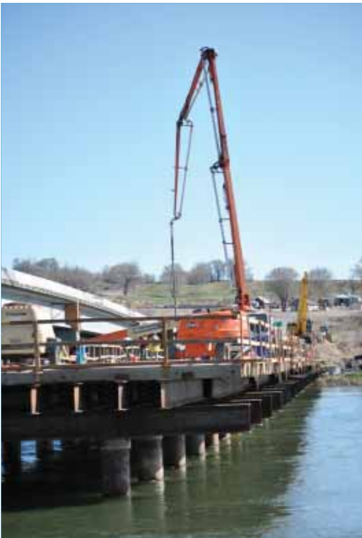
While much of the Owyhee County workforce has been told to stay home, Wadsworth Brothers Construction keeps working on the Snake River bridge in Marsing.
