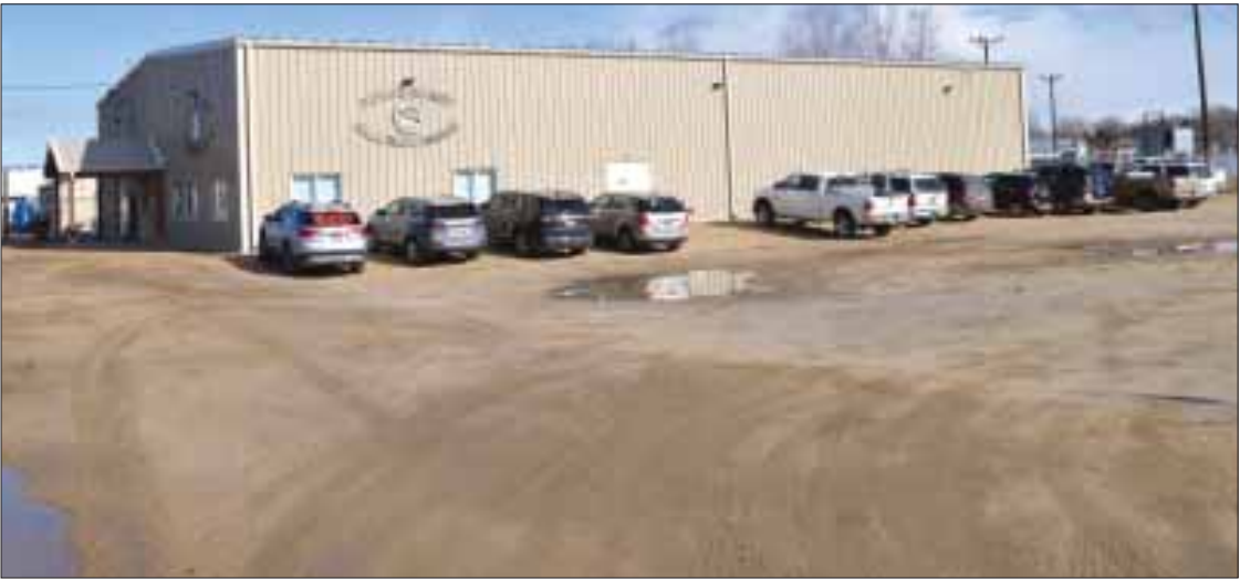
Owyhee County is working on a plan to pave the parking lot for the new community center at the fairgrounds in Homedale. Lincoln Day attendees had to dodge mud and puddles Monday.
