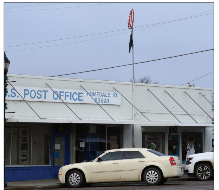
Strong winds blew the post office's U.S. flag over the pole.
