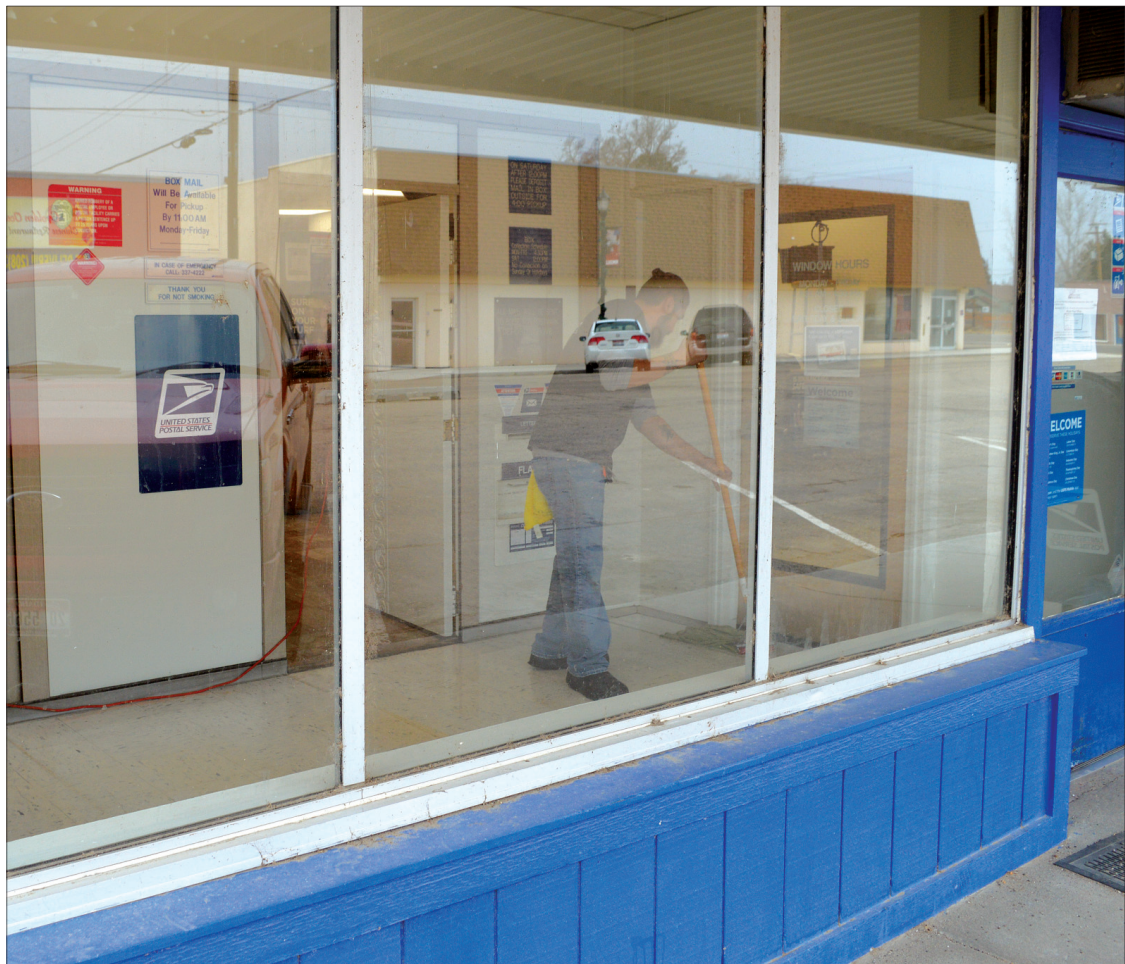
An employee of Caldwell-based Bob Howard Building Maintenance mops the new floor inside the Homedale Post Office on Jan. 21. The post office opens Monday after a 113-day closure.
