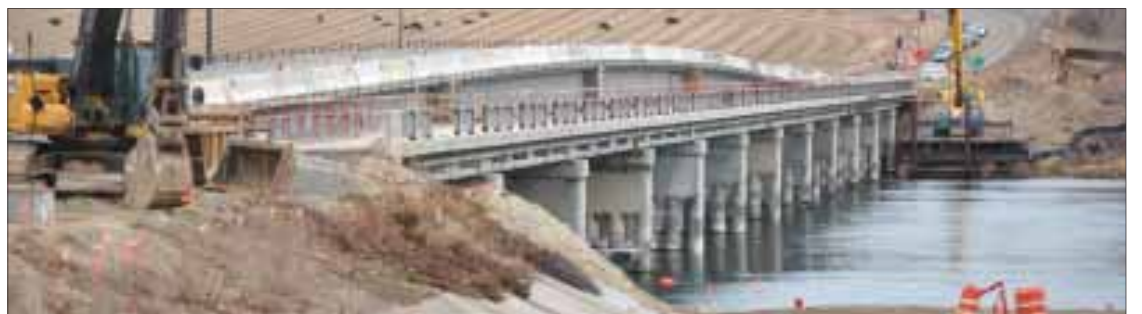
The new span arches to the north of the old Snake River bridge in Marsing.
