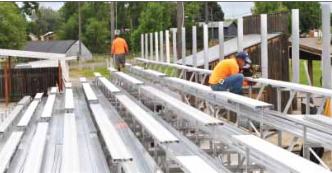
July: New fairgrounds bleachers The Owyhee County Rodeo Arena's much-needed upgrade — replacement of the covered grandstand bleachers — was completed in time for the Homedale Lions Club Fourth of July Demolition Derby.
