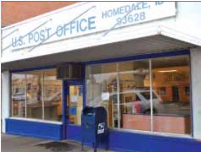
The Homedale Post Office closed for repairs in mid-October. Work hasn’t begun yet.
