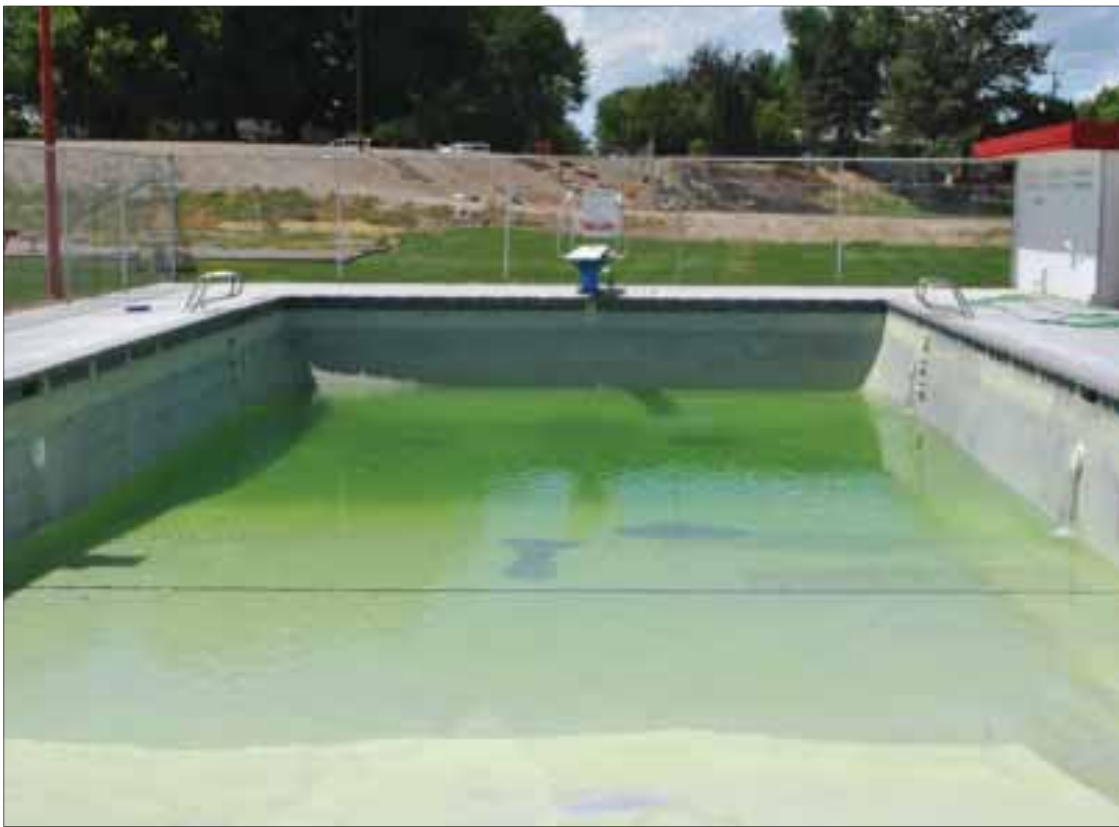
Left: Three cracks were discovered on the gunite floor for the Homedale City Swimming Pool, factoring into the delay of the facility's 2018 opening. Photo by Dave Downum. Right: Dark spots under the water show where patches were made as the pool fills Monday.
