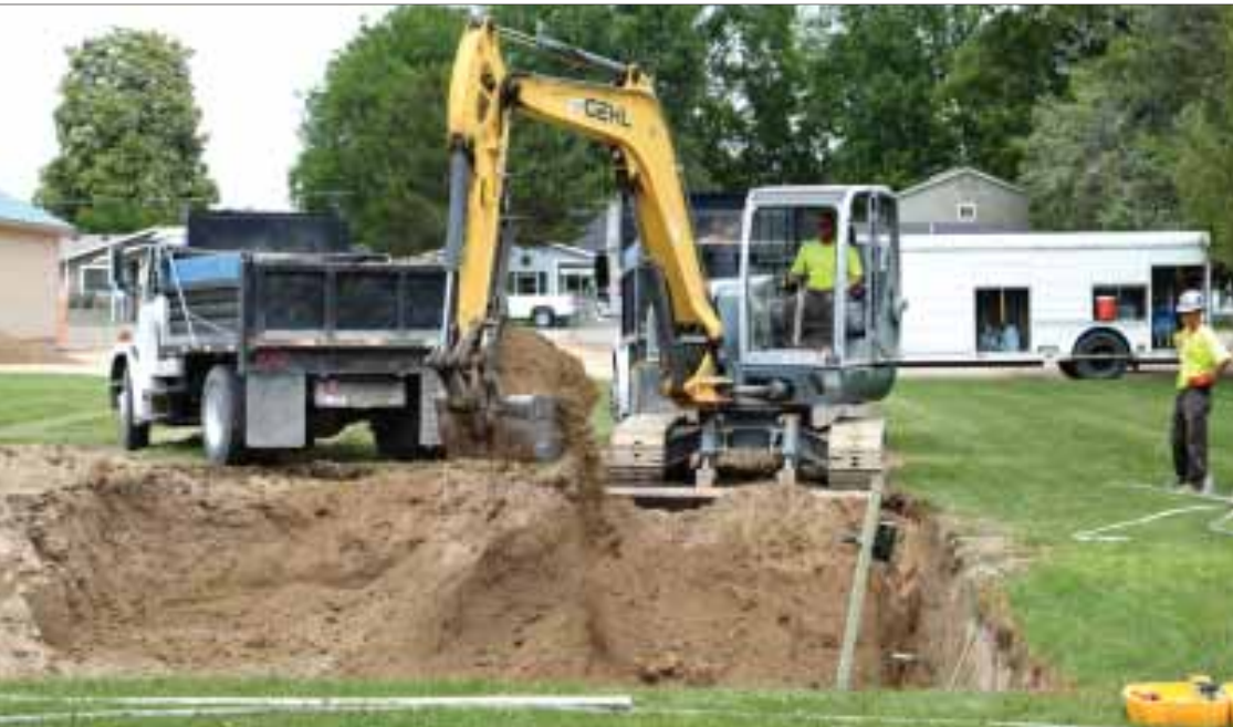
Duane Blankenship digs a seepage bed at Homedale Elementary School while Bricon Excavation co-worker Leif Bowman looks on Thursday.
